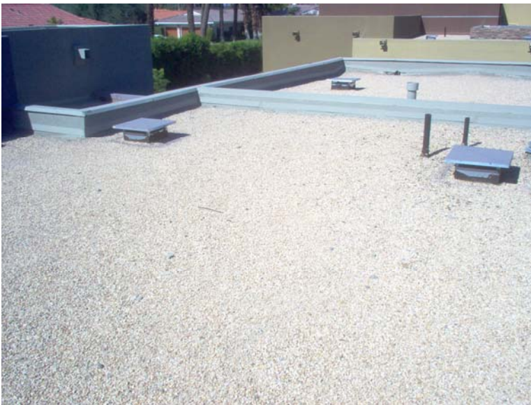
Another roof view.
