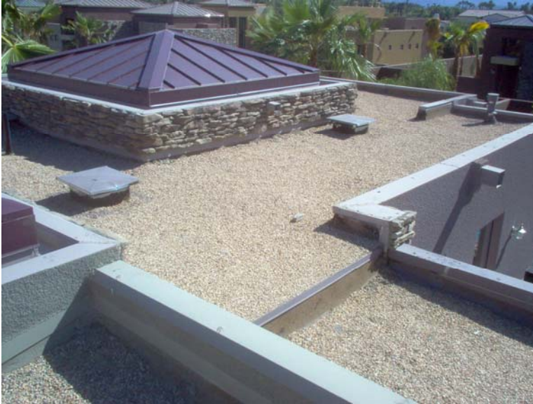
Typical roof view.
